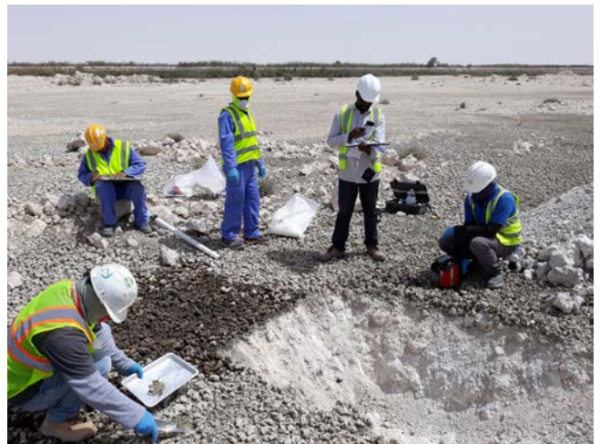
SUEZ monitoring TPH in-situ
