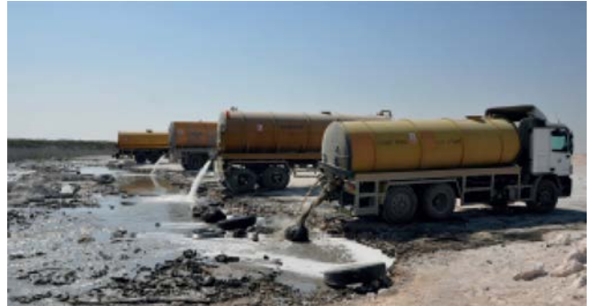
Tankers discharging wastewater into lagoons
